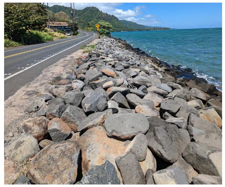
Engineered, uncemented rock revetments such as this may provide temporary protection and stability to sections of Kamehameha Hwy in windawrd O'ahu
